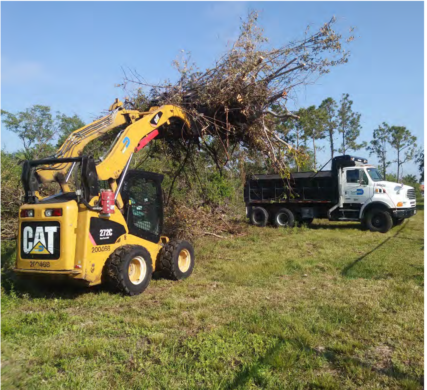
Figure 5. Miami-Dade County NAM hauling debris, Florida City Pineland, March 2018.
